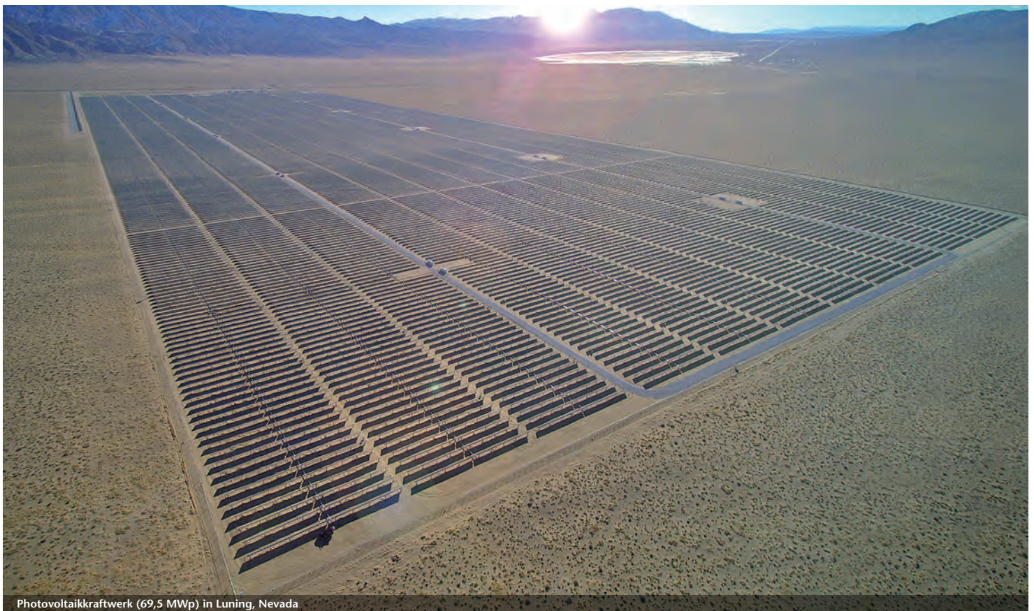
Photovoltaikkraftwerk (69,5 MWp) in Luning, Nevada
